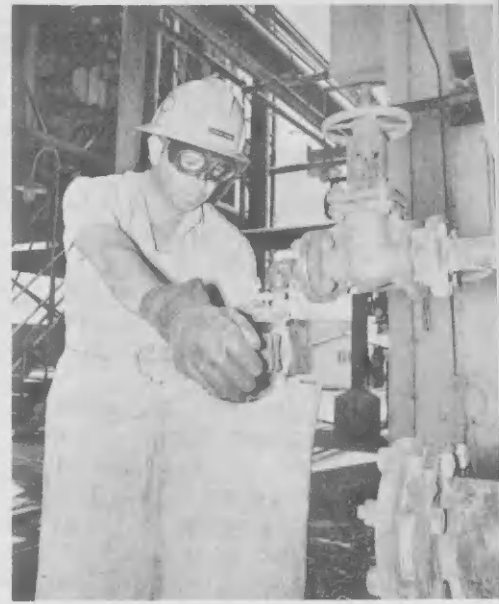
Juan Maduro wears chemical splash goggle against possible splashes when taking acid samples at the Acid Plant.
